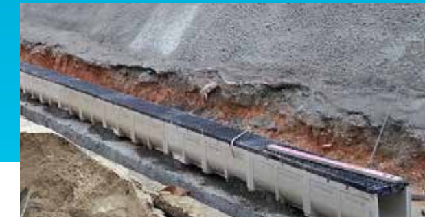
Supply & Install Precast Channel Mould
